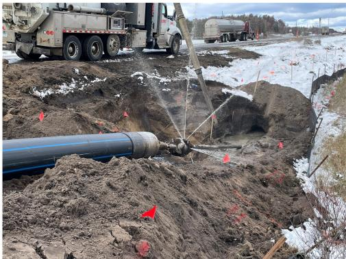
Photo #5: Pulling the first section of force main pipe back through the bored hole - Nov 2, 2023, 7:04 PM
