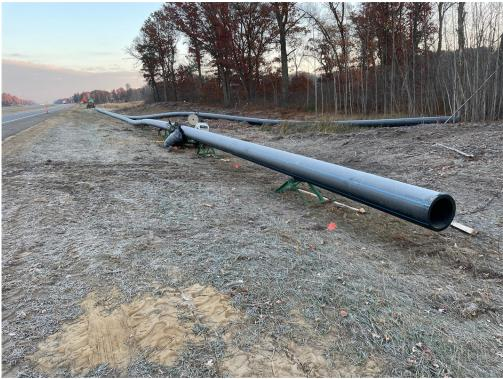
Photo #1: Fused carrier pipe along Highway 10 - Oct 30, 2023, 8:14 AM
