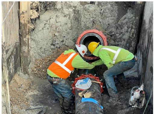
Photo #8: Working to connect the two sections of bored force main along Highway 10 - Nov 3, 2023, 11:22 AM
